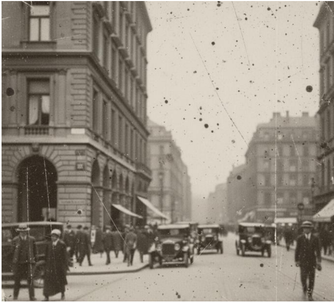
Fig.4. Damaged Input Image
